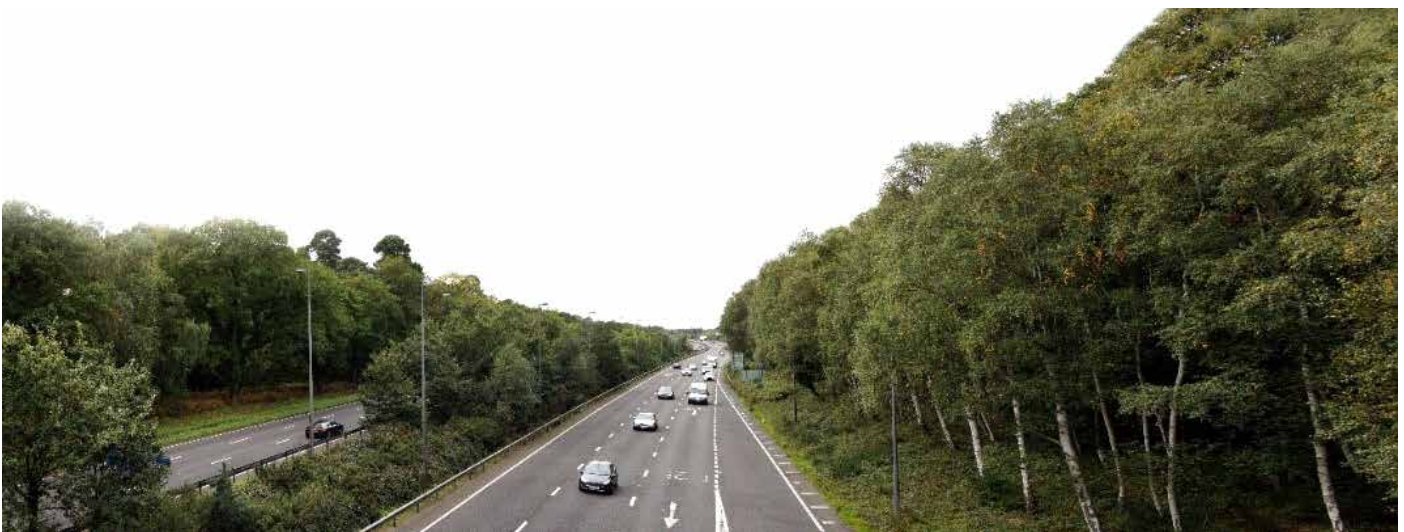
View southwest from Elm Lane footbridge towards Ockham Park junction, with Wisley Common woodland to the left, the wide vegetated central reserve, and the wooded cutting slope along the edge of RHS Wisley to the right
