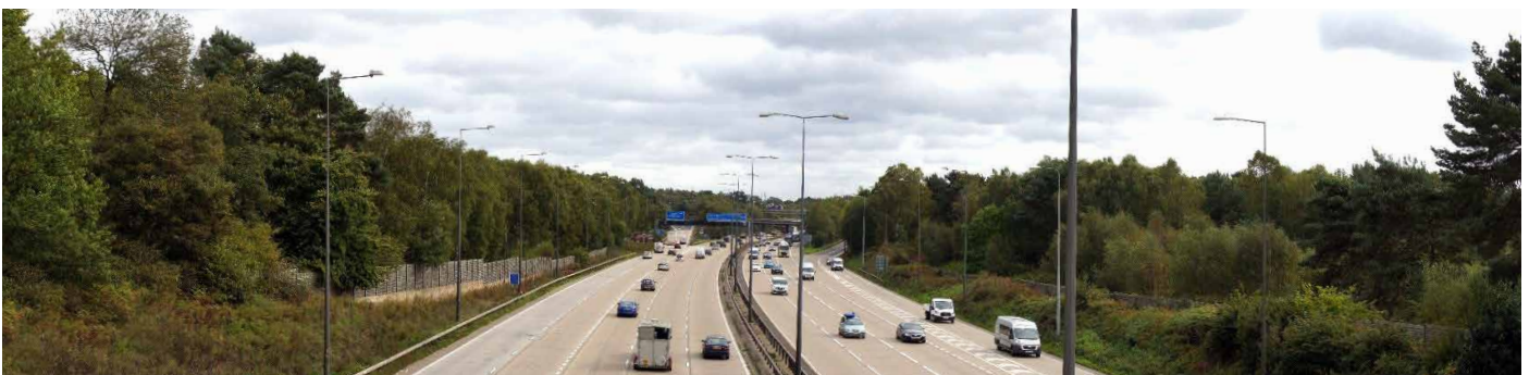
View west from Clearmount bridge towards junction 10, with noise barriers along the wooded edges of Wisley Common
